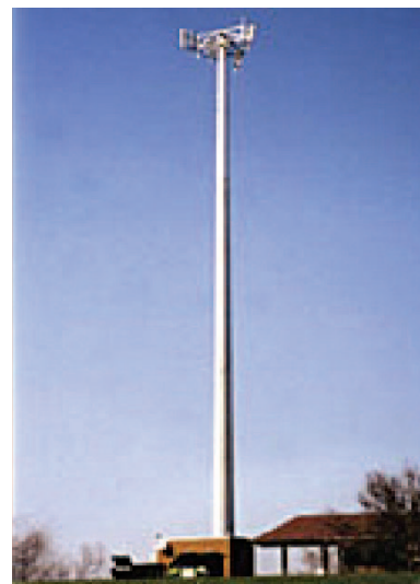
Figure 10: The application of the 100% solids rigid aliphatic polyurethane on a galvanized steel communication tower.
