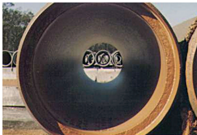
Figure 9: The application of a 100% solids elastomeric polyurethane system (both ceramic and anti-microbial modified), for a wastewater pipeline project involving the lining for 4,000' long, 72" diameter-size concrete pipes.
